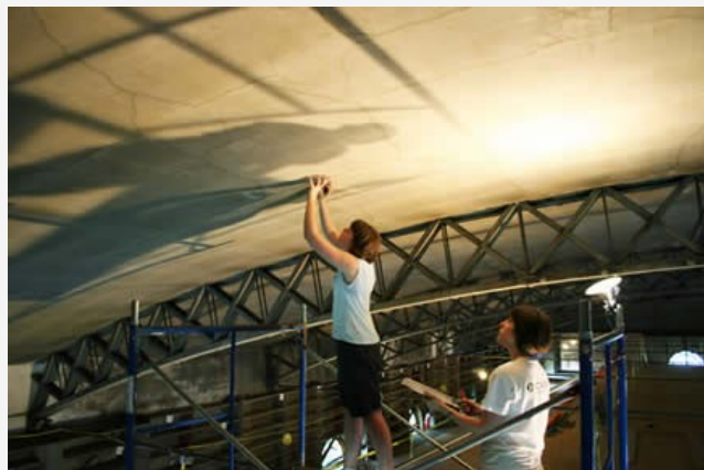
Marlene Goeke surveys the Wagner Free Institute's exhibit hall ceiling.
